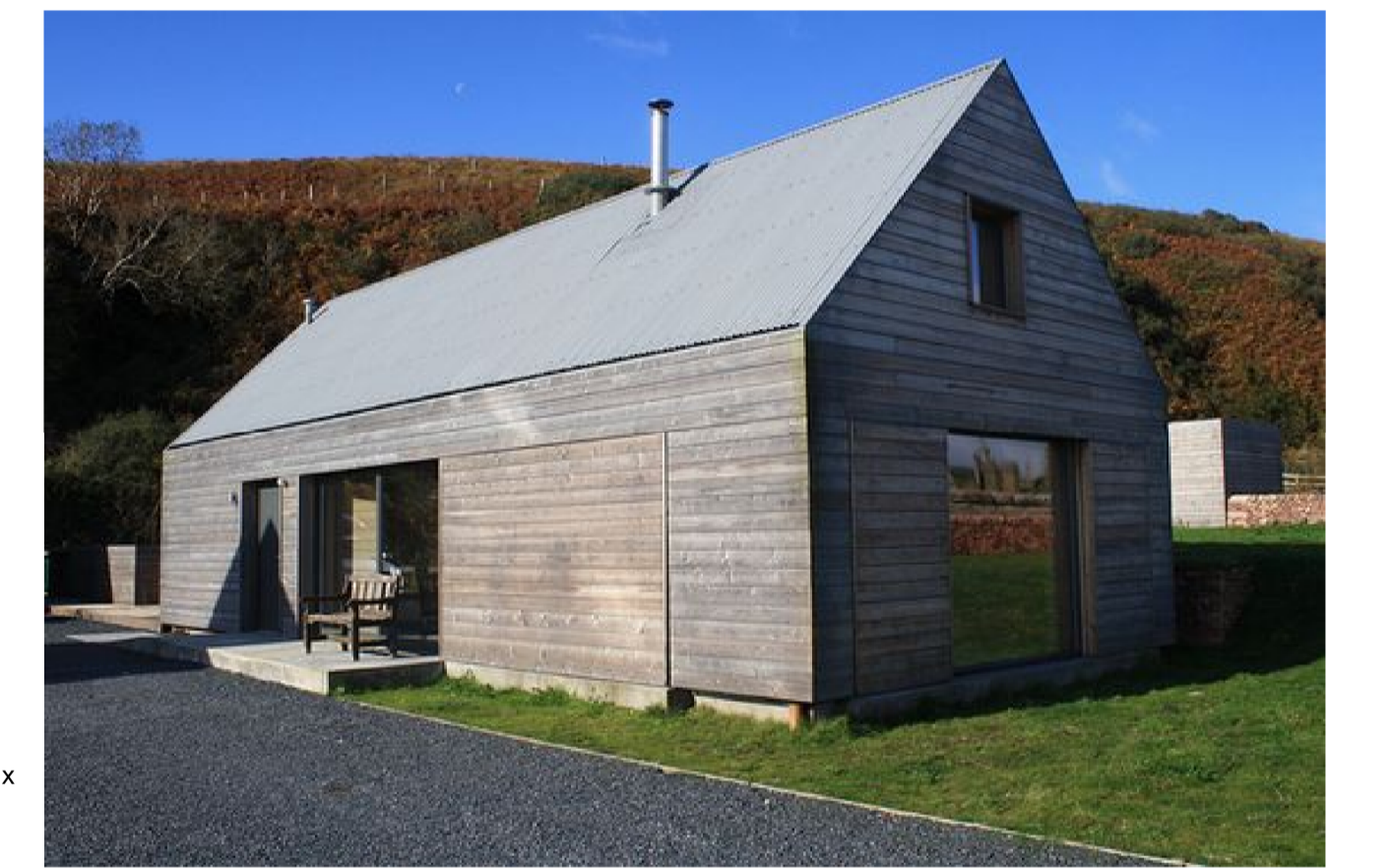
Timber cladding with corrugated metal roof
